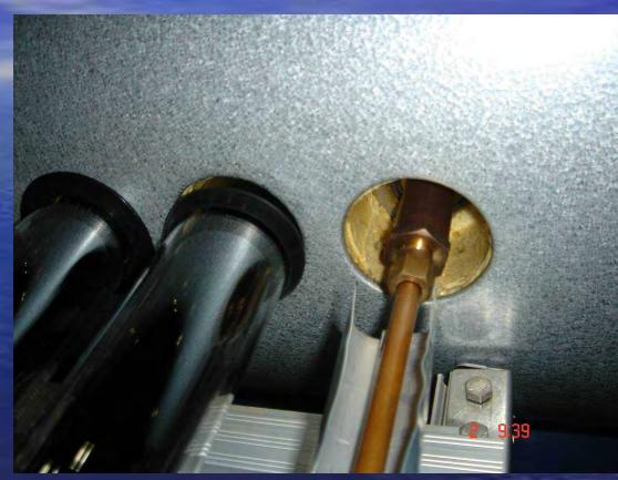
Hot condenser end of heat pipe into cold water flow Plate end of heat pipe with chrome for corrosion protection
