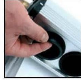
8. Install the anti-dust circles (It's better to smear some soap liquid, so it can lubricate when install vacuum tubes)
