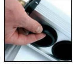
12. Turn solar collector back and install anti-dust circles
